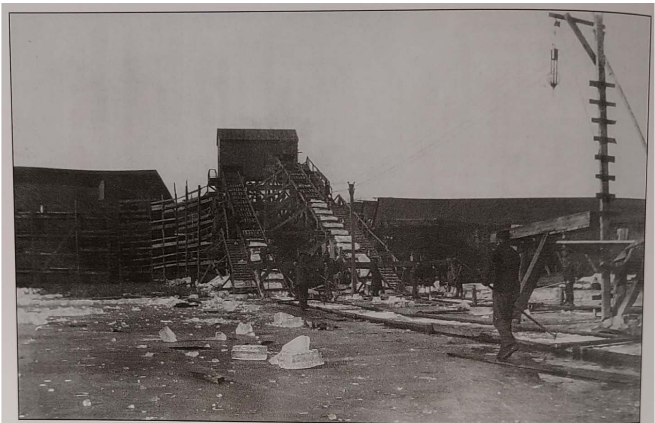
These elevators sat on the lake's northern edge in Armour Town in 1910. Ice blocks rode up the elevator and into the barn, where a man with an ice hook pushed the blocks into orderly rows. When the floor was covered with ice, the ice was covered with sawdust, marsh grass, or cattails and another layer of ice was placed on top. This process was repeated until the barns were full. (LRCM.)
